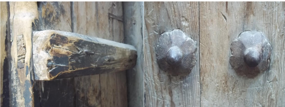
Fig.8: Pictures of decorative nail made by a local blacksmith is hammered from the outside, and after passing through the boards and support wood, it is bent.
