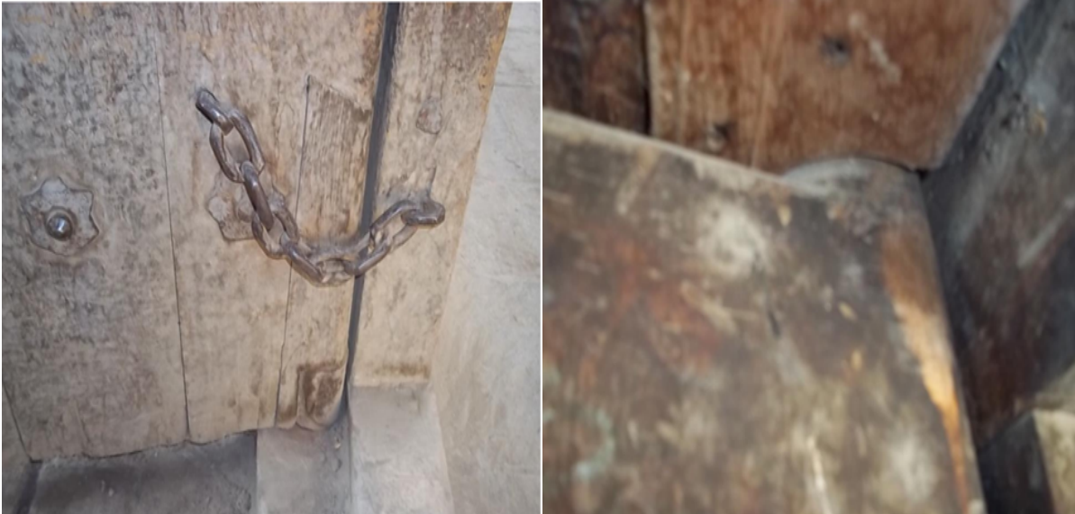
Fig. 7: Pictures of ball bearing door panel at lower and upper connection
