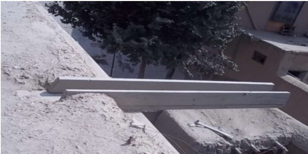
Fig.5: A picture of wooden gutter of roof
