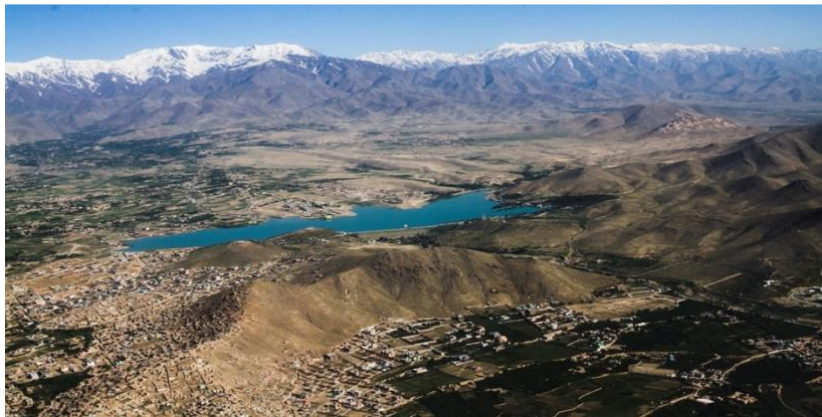
Figure . Qargha Dam and Reservoir in Kabul Province
