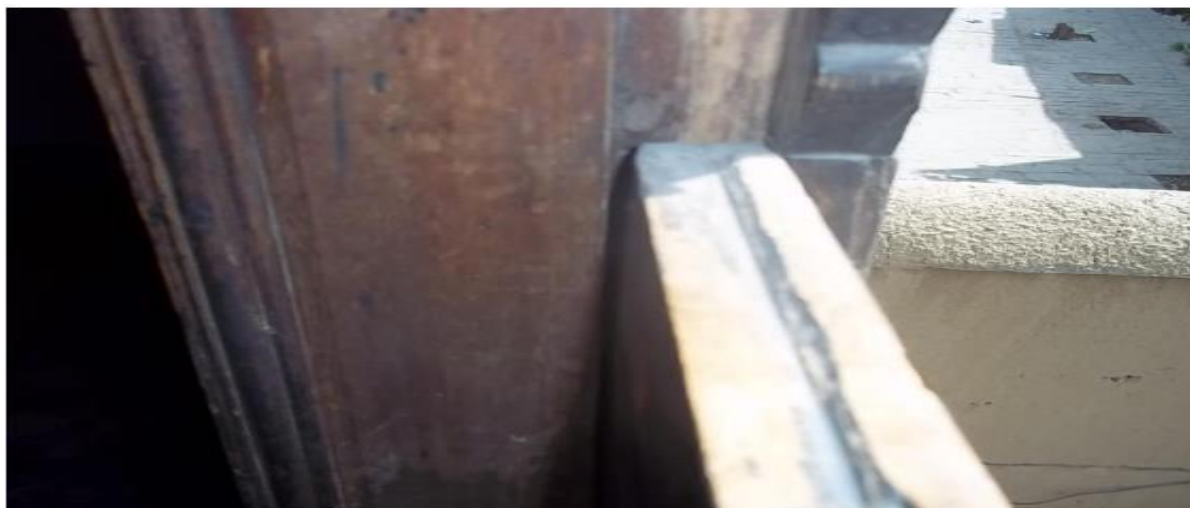
Fig.2 - The image of one of the parts with a layer of wooden boards that has depression in the middle
