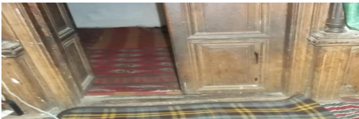
Fig.8 - Photo of the hallway (day room) door (Double leaves)
