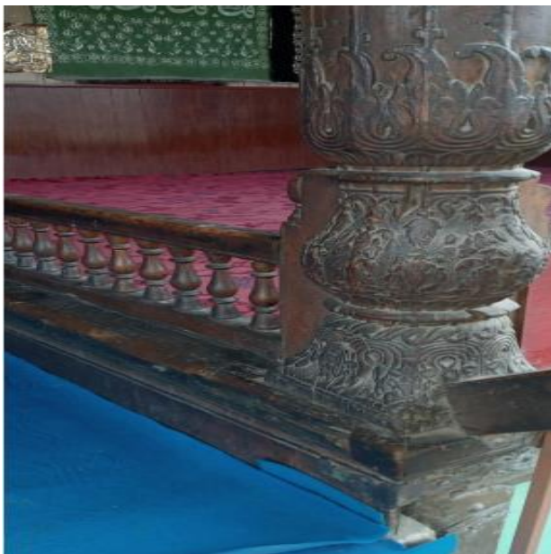
An image of the woodwork decoration of the covered veranda
