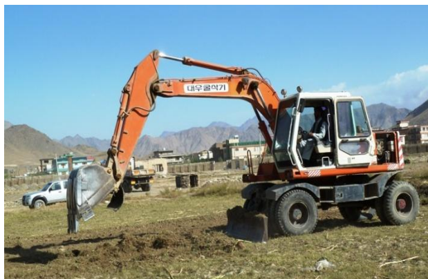
Excavation work at Rishkhur, Kabul, June, 2012.
