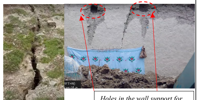
new crack in the ground
