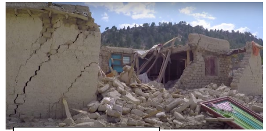
Cracks in a wall
