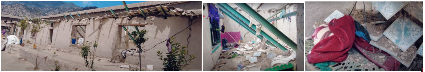
The steel I beams that supported the ceiling floor above look intact, but separated from the supporting wall that probably had less supporting edge at the opposite wall, and brought the ceiling floor down
