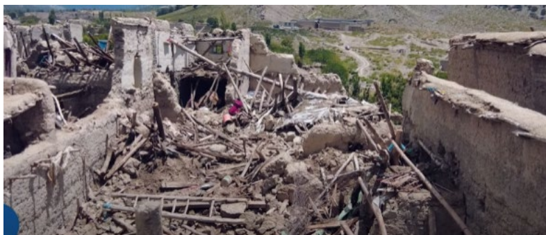
House collapsed completely
