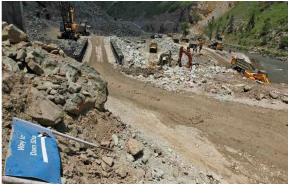
Figure 4. Shatoot Dam under construction at Tangi Saidan
