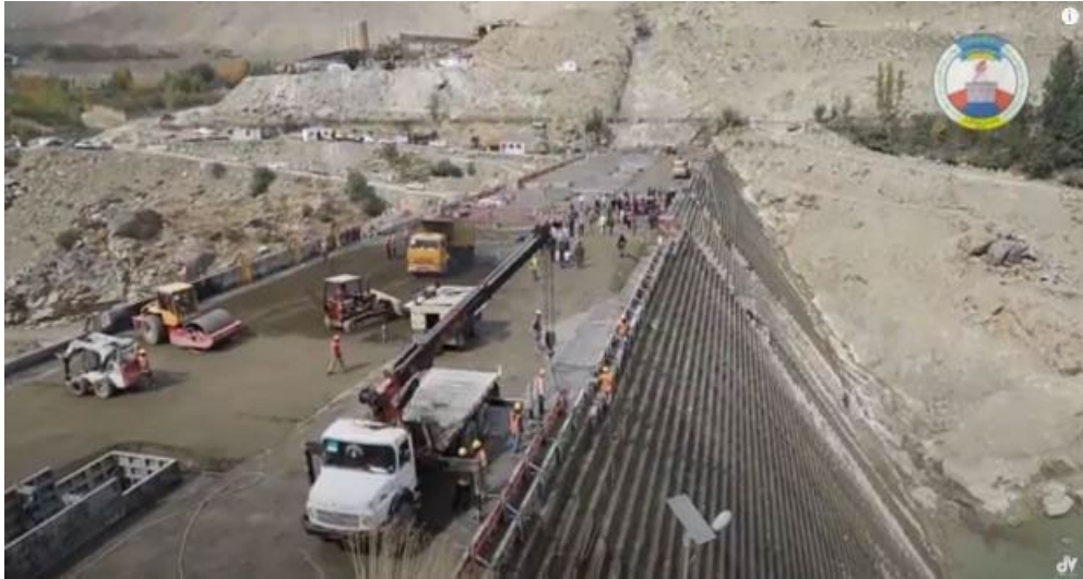
Figure 1. Shah-wa-Arus Dam under construction
