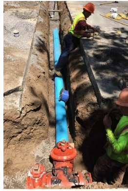
Figure 7: Underground Piping Project- Replacement of Water Mains
