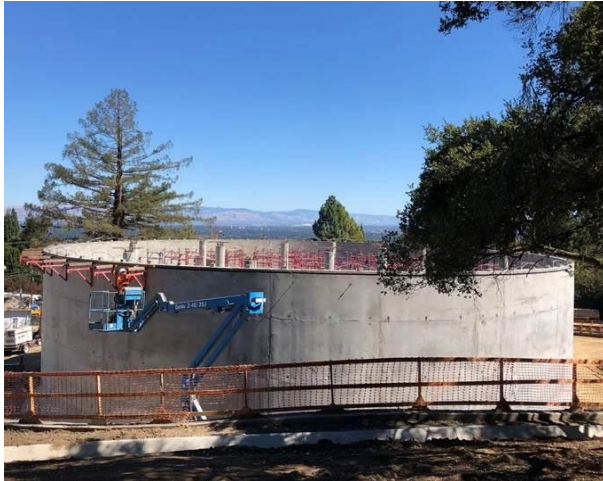
Figure 6: Construction of Water Tank in Redwood City, CA
