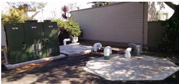
Figure 9: Sanitary Sewer Pump Station in Redwood City, CA
