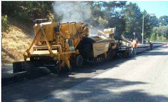
Figure 3: Asphalt Overlay Construction
