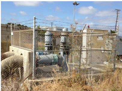
Figure 8: Storm Drain Pump System in Redwood City, CA
