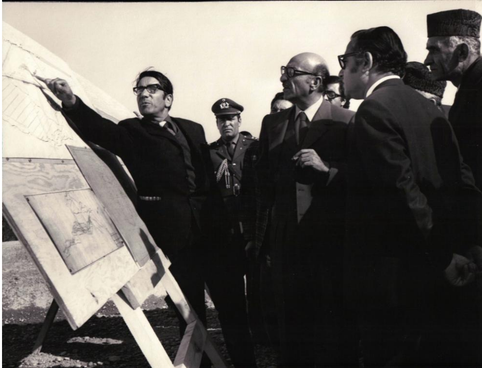
Engineer Aman (left) showing work progress to King Zahir Shah (center) and Governor Mir Akbar Reza (foreground) during the early 1970s.
