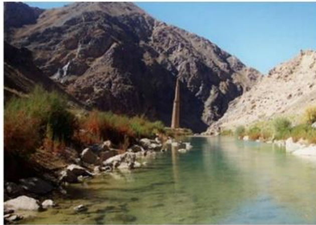
Figure 3 example of foundation settlement – Jam Minaret in Ghore Province of Afghanistan
