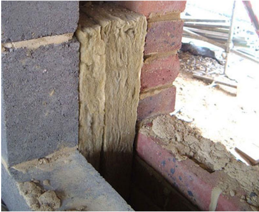
Figure 3 – Fiberglass as wall insulation reduces and minimizes heat loss in winter and prevents heat gain in summertime through walls and simultaneously, prevents sound transmission inside and outside the building.
