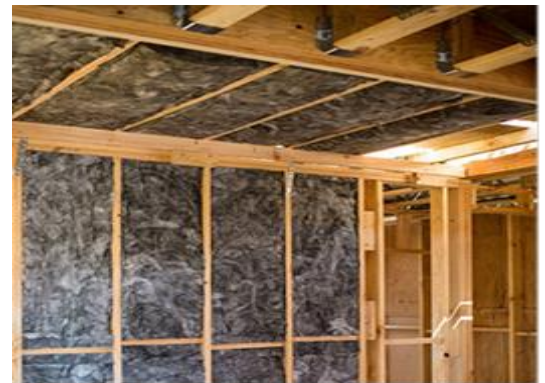
Figure 2- Fiberglass insulation in wall
