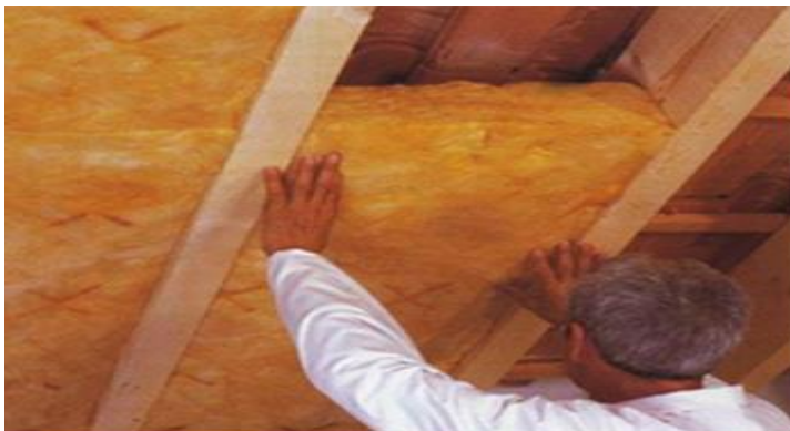
Figure 1- Fiberglass insulation in ceiling
