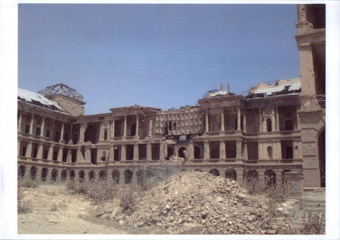
View from the Yard (Southern view) of the ruins of historic Palace of Dar-ul-Aman
