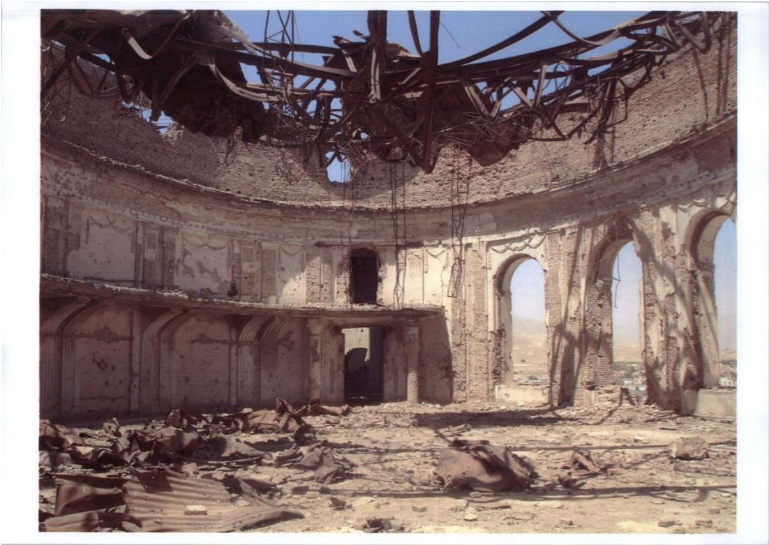
Plenary Hall view of the ruins of historic Palace of Dar-ul-Aman
