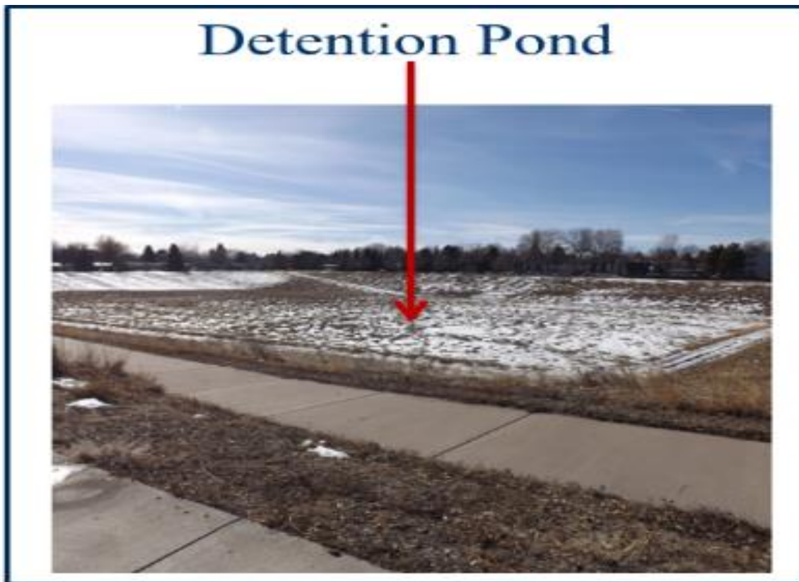
Figure 5. Stormwater detention pond to store temporary excess storm runoff from the upstream development and release it slowly at historic flow rate.
