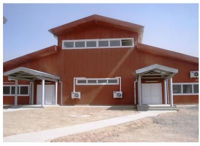
Using prefabricated steel panels, Ti designed and built this modern kitchen and dining hall for a facility that serves up to 500 personnel.
