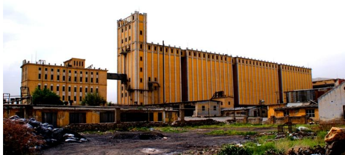
Kabul Silo main storage and the mill
