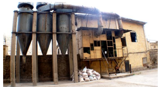
Kabul Silo Grain Intake building
